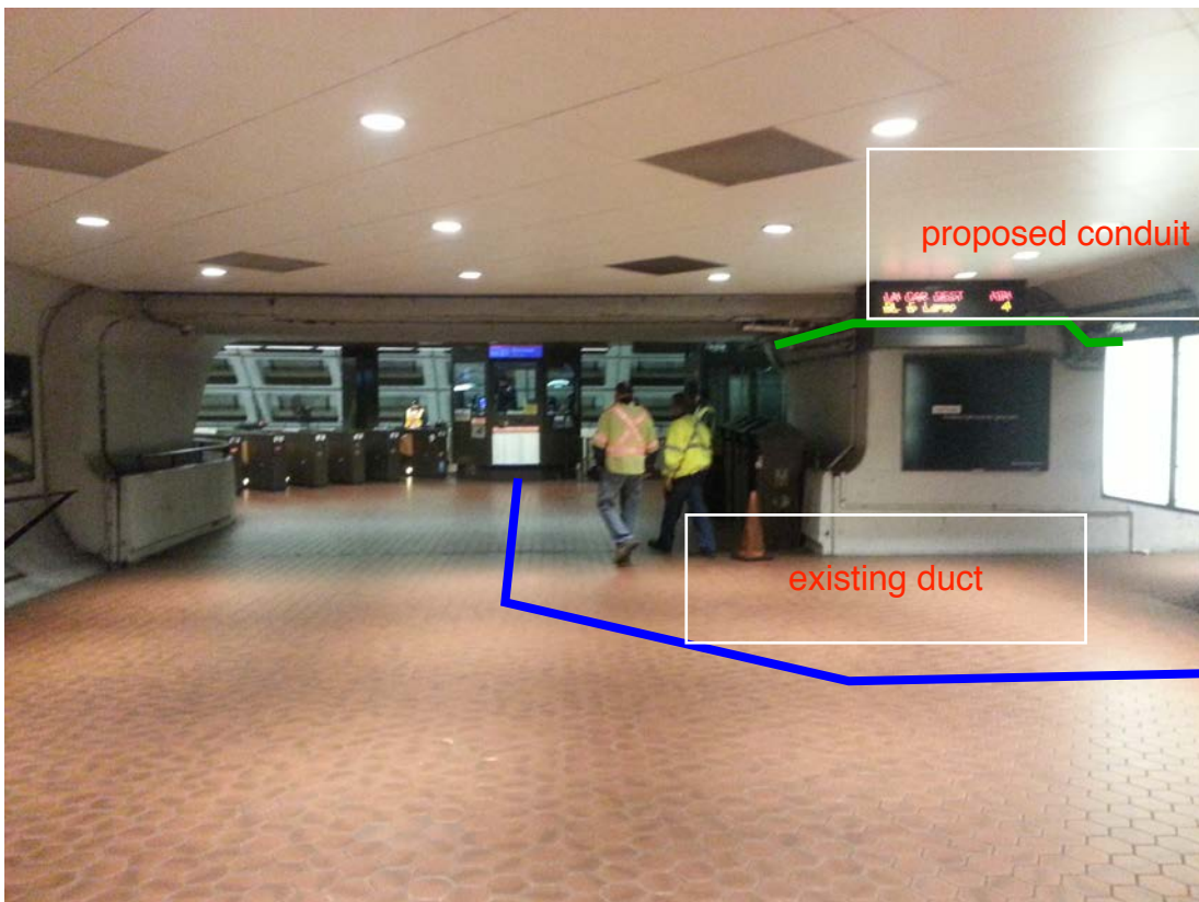
Photo #2 – D05 Capitol South: Proposed overhead conduit and existing in floor duct runs
