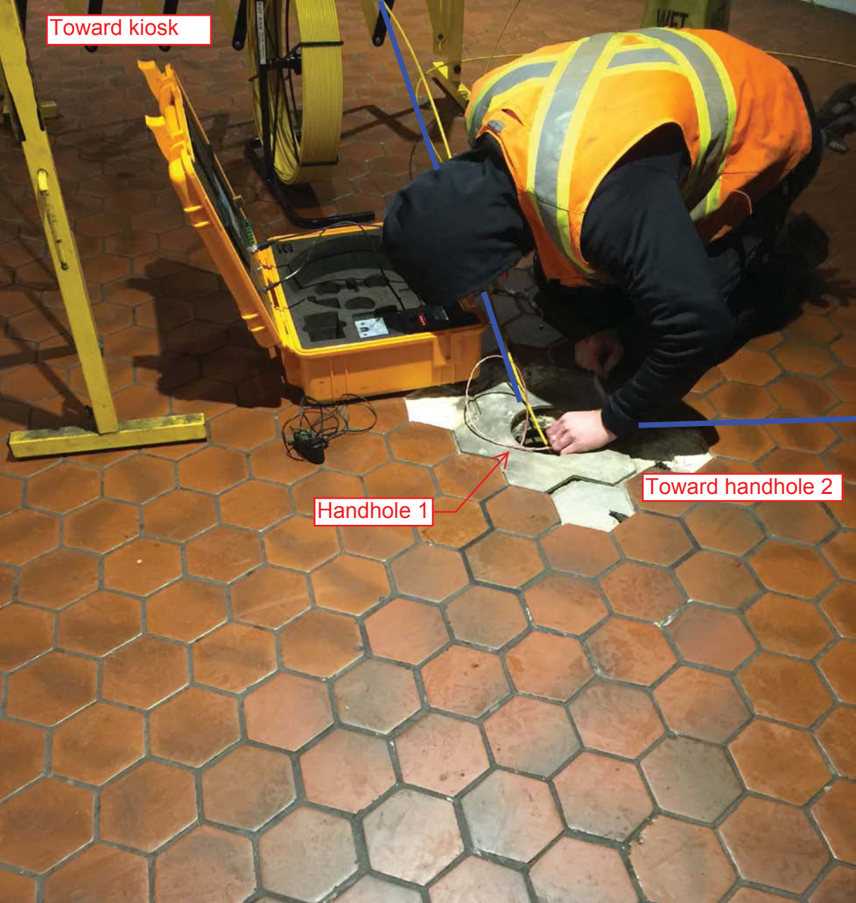
Picture 4: D06 Eastern Market – Handhole 1 location exposed
