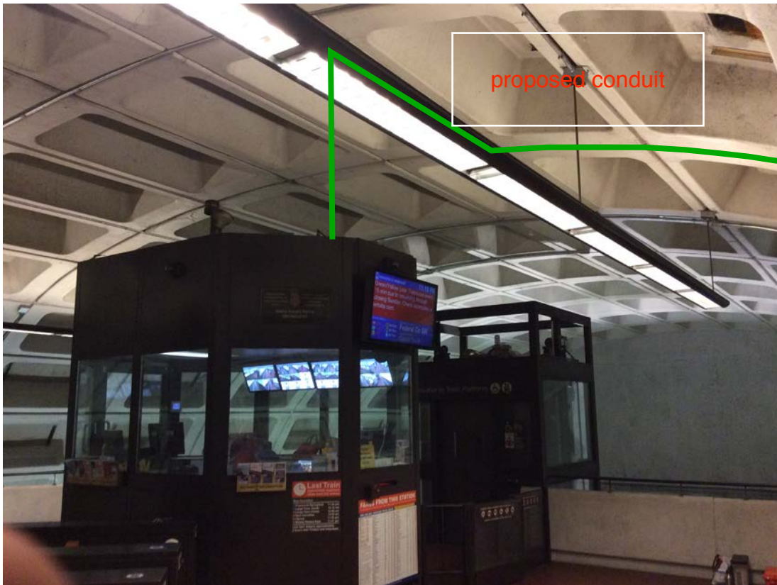
Photo #2 – D05 Capitol South: Proposed overhead conduit and existing in floor duct runs
